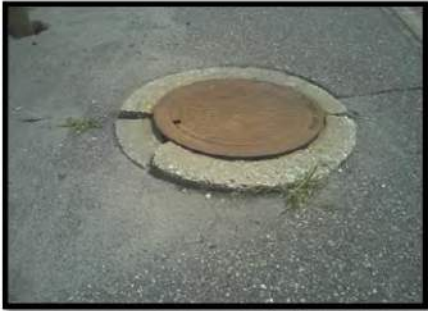
Traffic Signal Handhole
