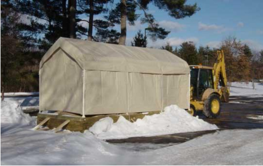
Salt stored in a small elevated and covered shed located on impervious surface.
