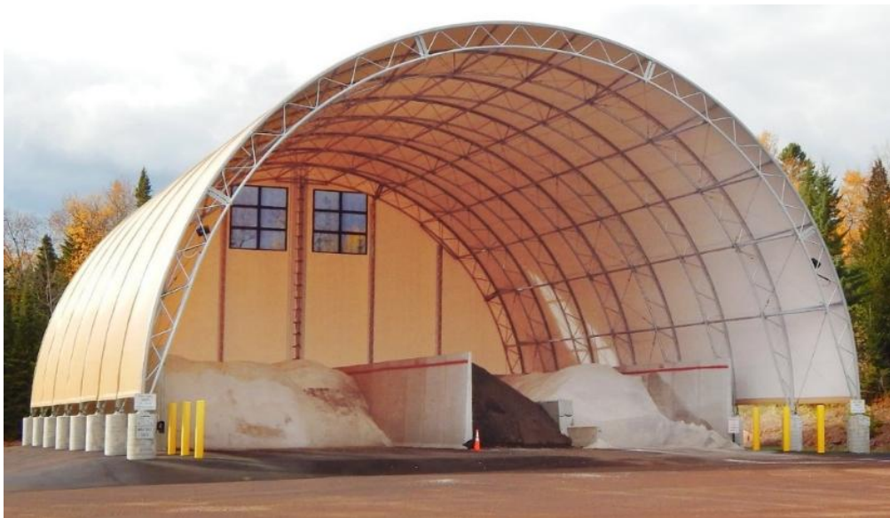
Salt stored in a covered building and on impervious surface.
