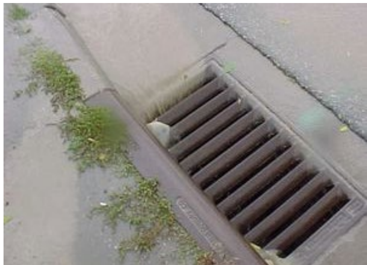
Stormwater entering a storm drain (Minnesota Stormwater Manual)
