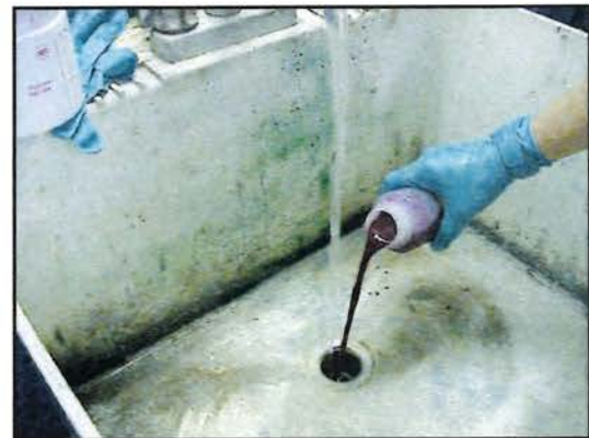
Figure 63: Dye Testing Plumbing (NEIWPCC, 2003)
